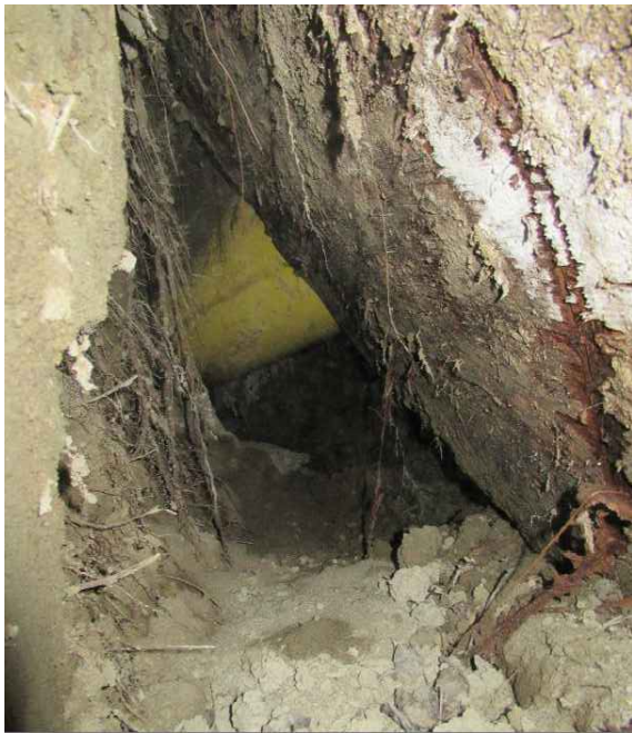
EXPOSED PIPE IN TENSION CRACK
