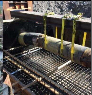
Photo 3: Installation of concrete form work for the base of the vault.
