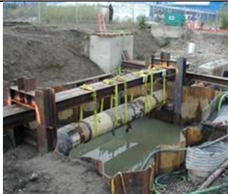
Photo 2: Dewatering of work area following the installation of the piling.
