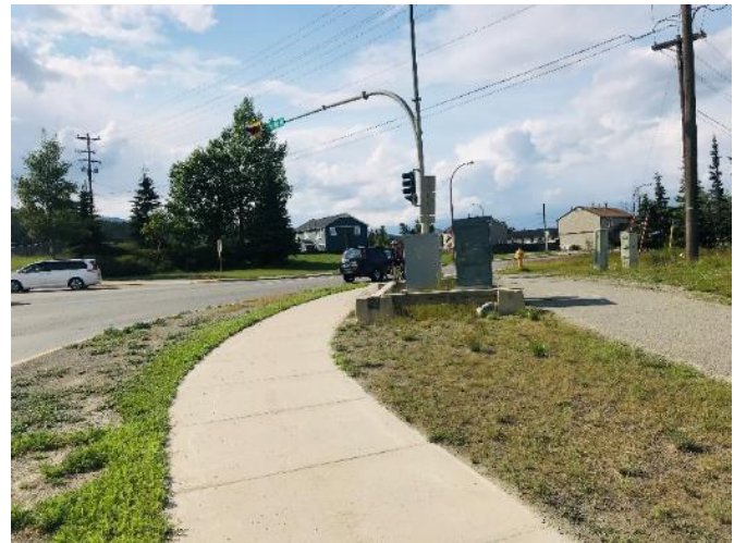
Figure 3-3 Conflicts due to Large Turning Radius and Visibility Obstruction
