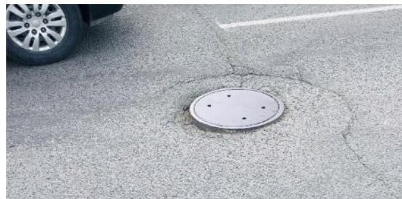
Figure 3-8 Pavement Level around the Utility Cover
