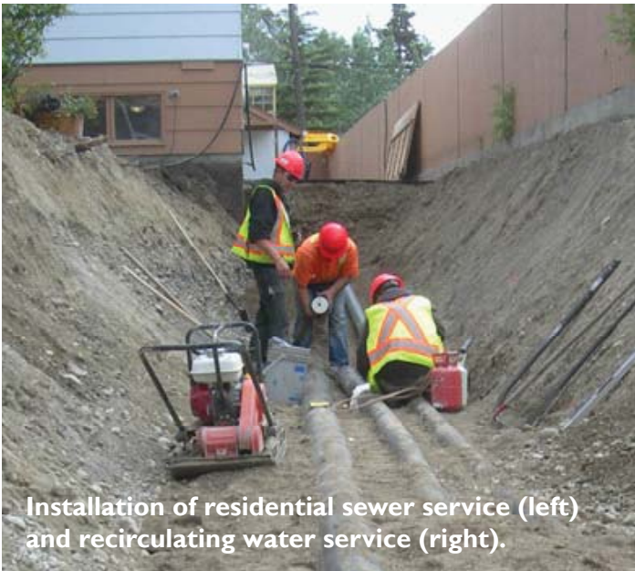
Subsurface works, 3 to 4 metres below grade.
