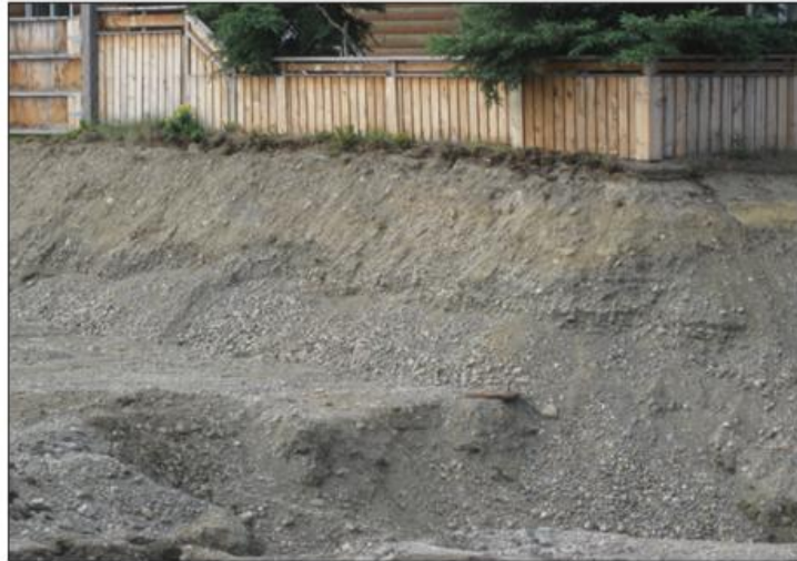
Figure 11. Fluvial sand and gravel exposed in infrastructure excavation near Wheeler St. and 6th Ave. This material underlies much of downtown Whitehorse, which is built on a terrace of the Yukon River (gsFt).
